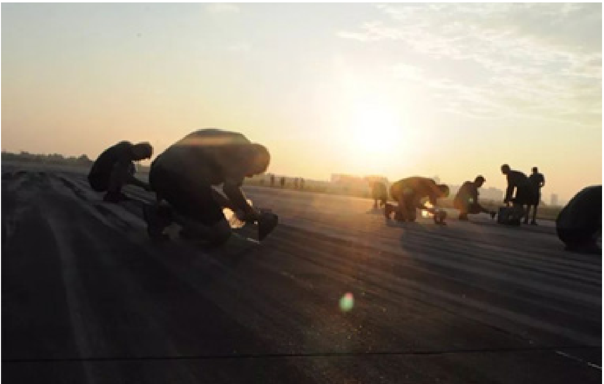
Airfield Services Company resealing runway after repairs 32
