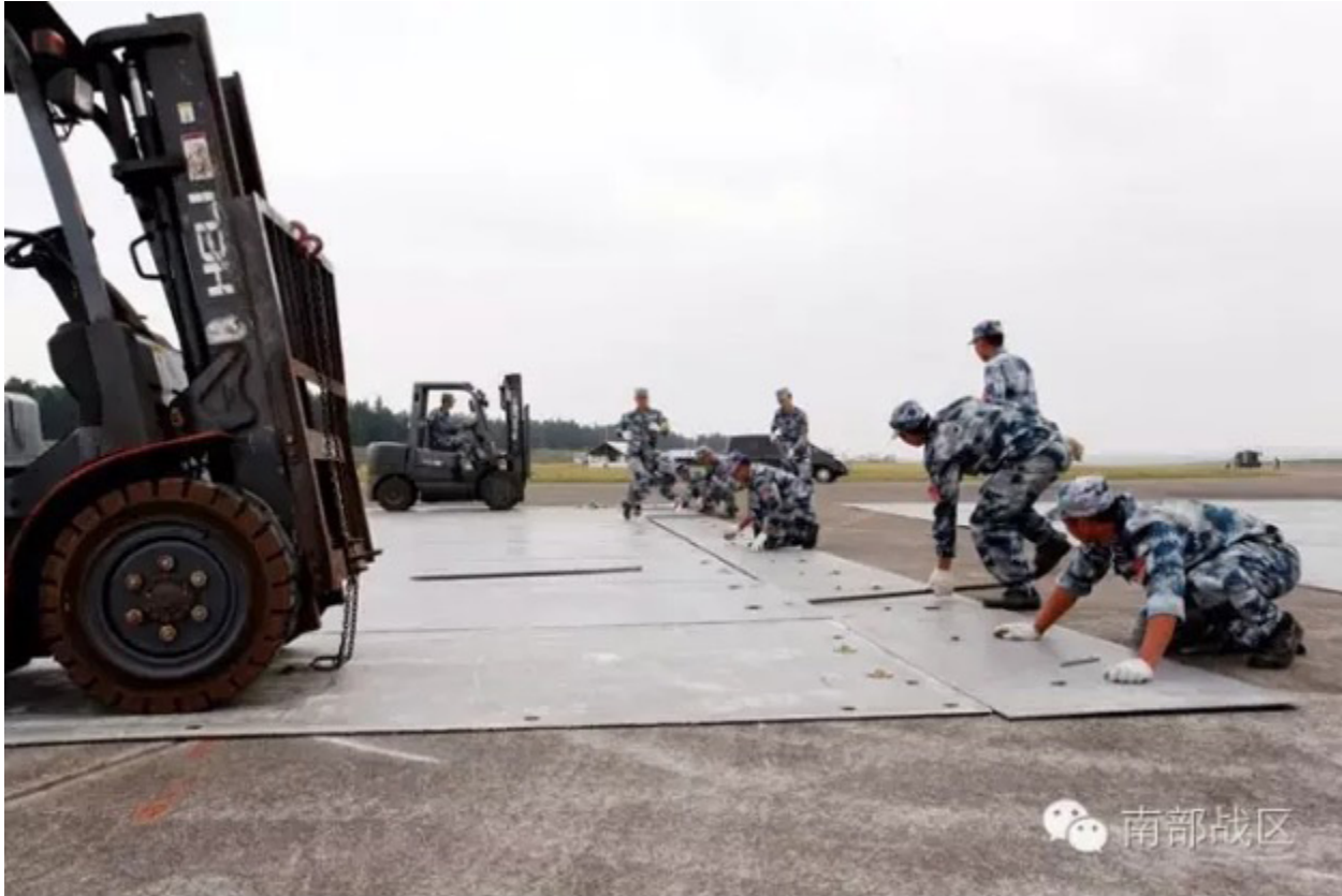
Militia laying steel plates over a damaged runway section 36
