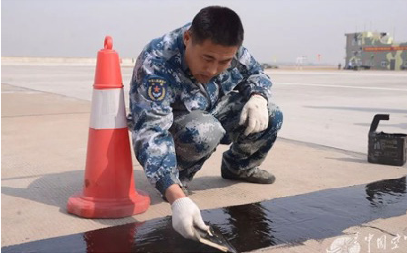
Airfield Services Company resealing runway after repairs 31
