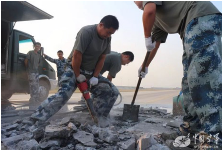
Airfield Services Company breaking up a damaged runway section 30
