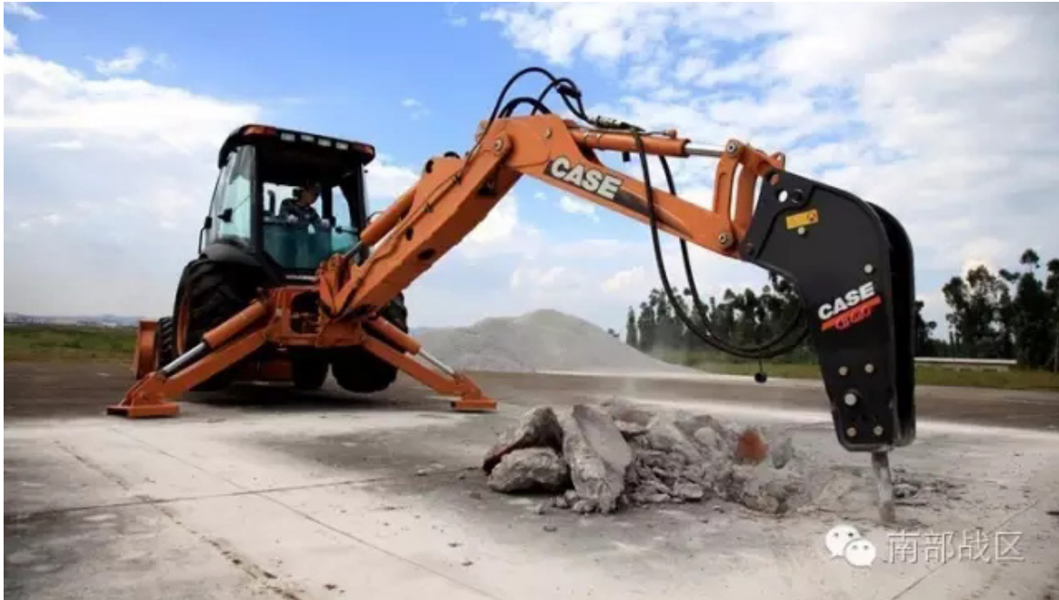
Civilian construction equipment used for runway repair 104
