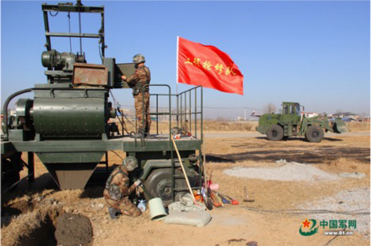
JLSF practicing refilling craters with concrete 39
